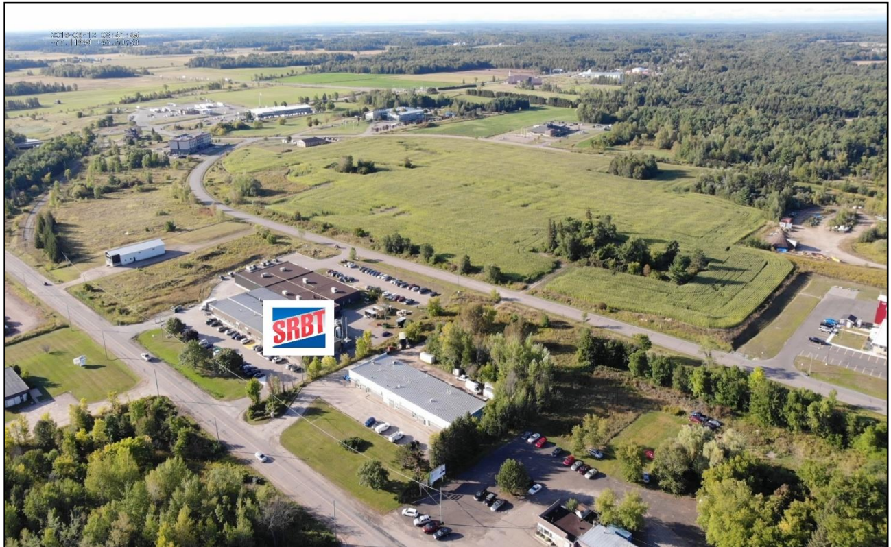
FIGURE 4: AERIAL PHOTOGRAPH LOOKING SOUTHWEST OF SRBT FACILITY
