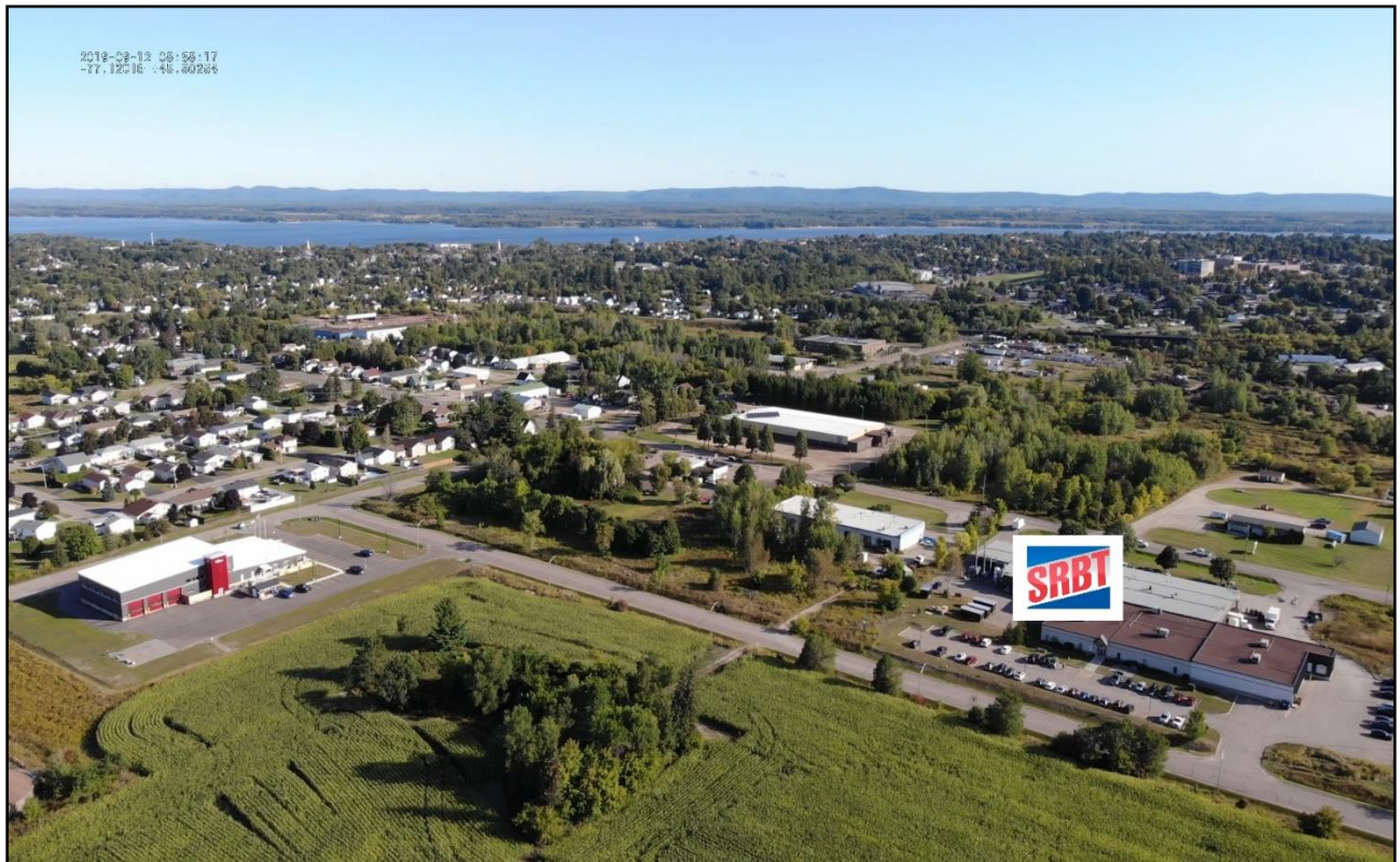
FIGURE 6: AERIAL PHOTOGRAPH LOOKING NORTHEAST OF SRBT FACILITY
