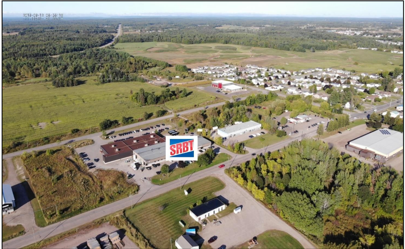
FIGURE 5: AERIAL PHOTOGRAPH LOOKING NORTHWEST OF SRBT FACILITY
